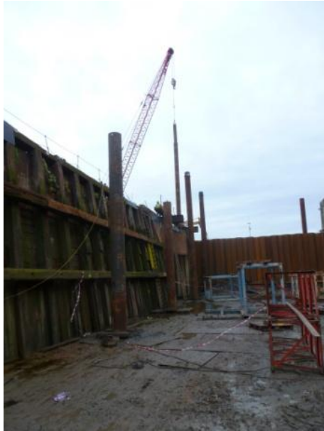
Extended 18-19mx475 bearing piles
