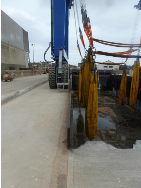
Testing the runways with water weights before the refurbished dock is flooded
