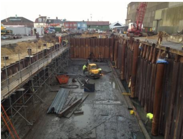
Both sides of dock faced with MX10 piles and left hand side ready to receive 610mm I beams
