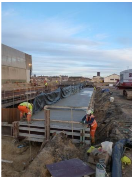
Screeding off 1 st beam
