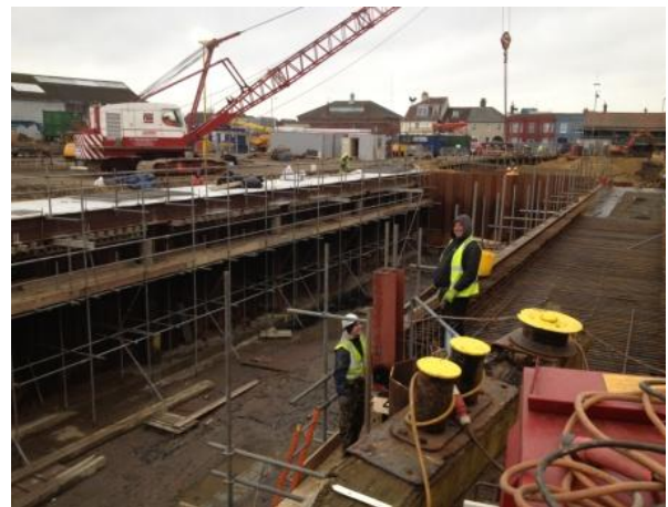
Preparing 2 nd beam
