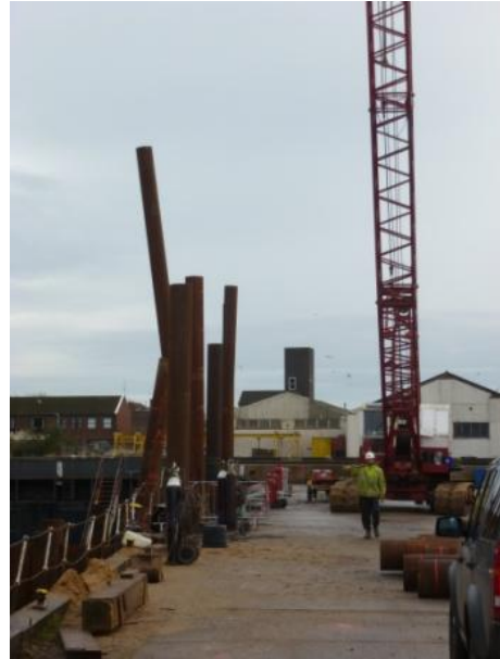
Back line of bearing piles and raker with extensions added before 2 nd drive
