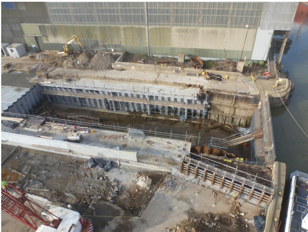
Ariel view of the boat hoist runway
