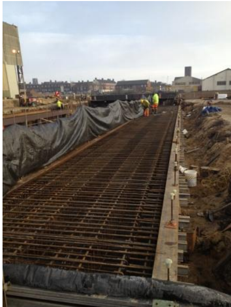
1 st runway 35mx3mx610mm with reinforcing steel installed
