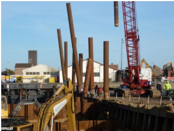
Back line of bearing piles and raker with extensions added before 2 nd drive
