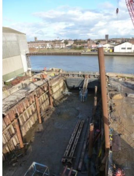
Ariel view of both sides of old dry dock with piles
