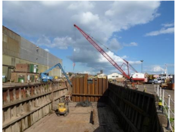
Installing sheet piled diaphragm wall 9m long PU12
